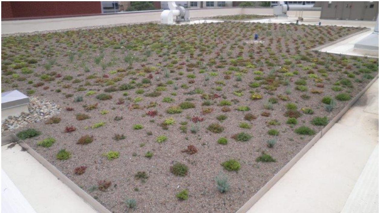
Olson Hall Roof Replacement – View looking southeast
