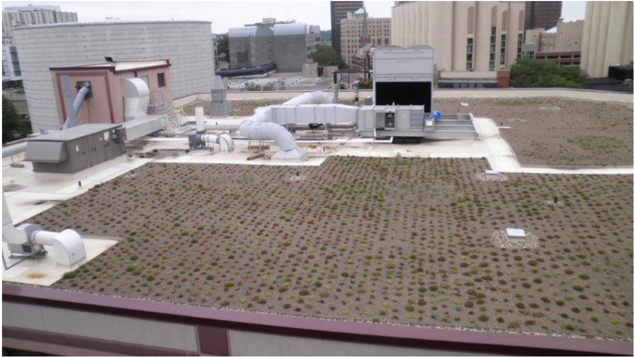
Olson Hall Roof Replacement – View looking west
