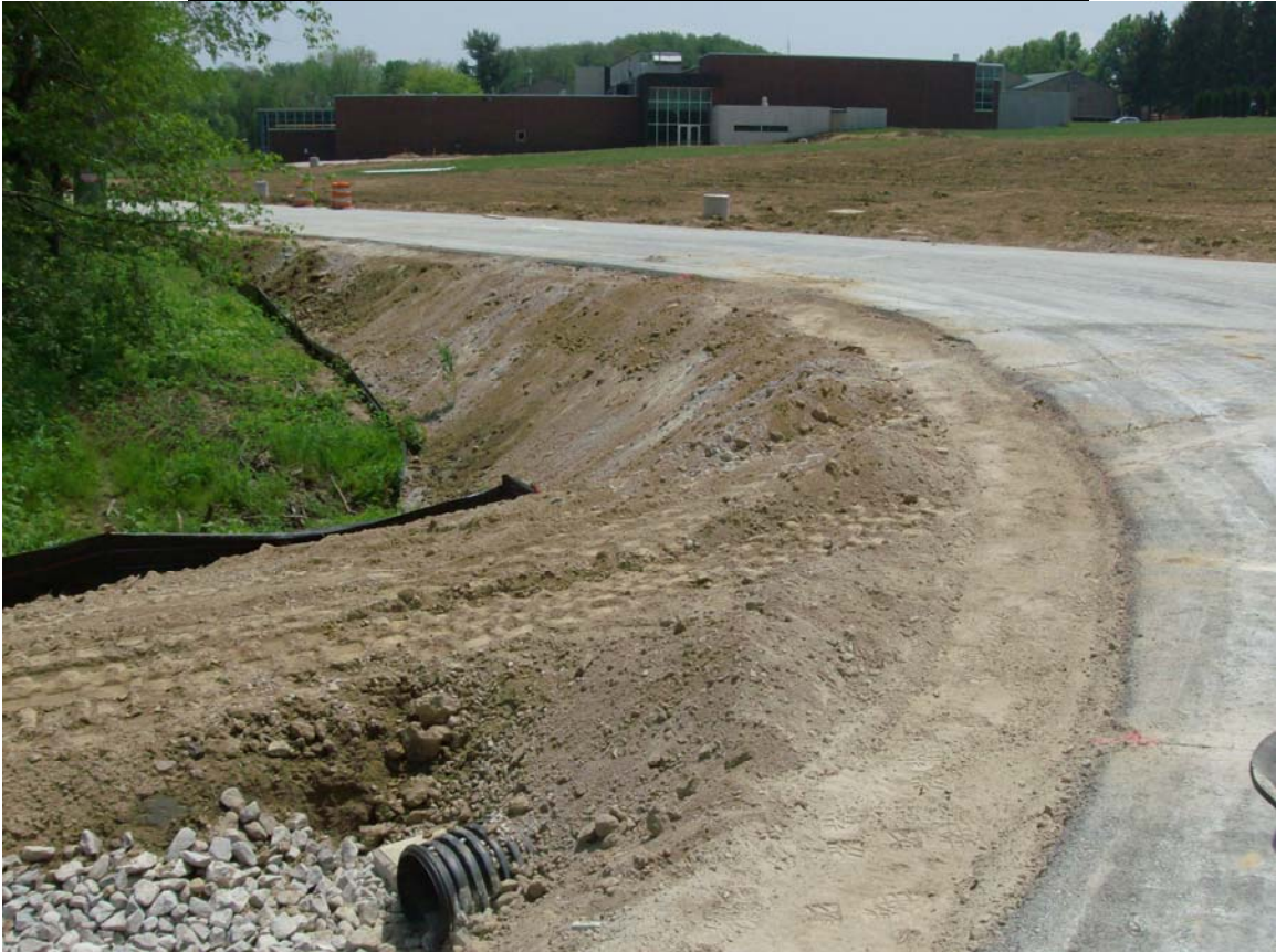
Wayne Campus North Entrance Drive – View looking West
